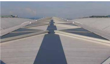
isting PVC sheet membrane waterproofing system of Terminal 1 roof. The loading of the additional waterproofing system to be imposed on the roof was not to exceed 2.5 kg/m², while its fixing system needed to satisfy the design wind pressure with the highest figure 8.5kPa. Moreover, seam welding was mostly done by handheld welding guns instead of automatic machines. This was due to the dome shape profile of the roof where automatic machine could not be implemented.
